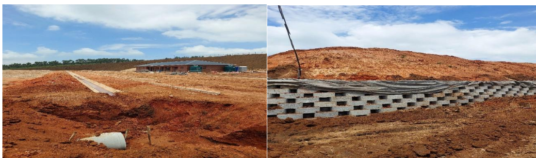
Photos: Construction of Hlokozi Sport field in Ward 6
