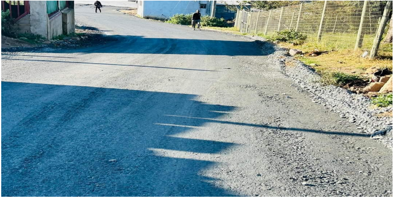
Photos: Construction of Old Clinic Asphalt Road Ward 10
