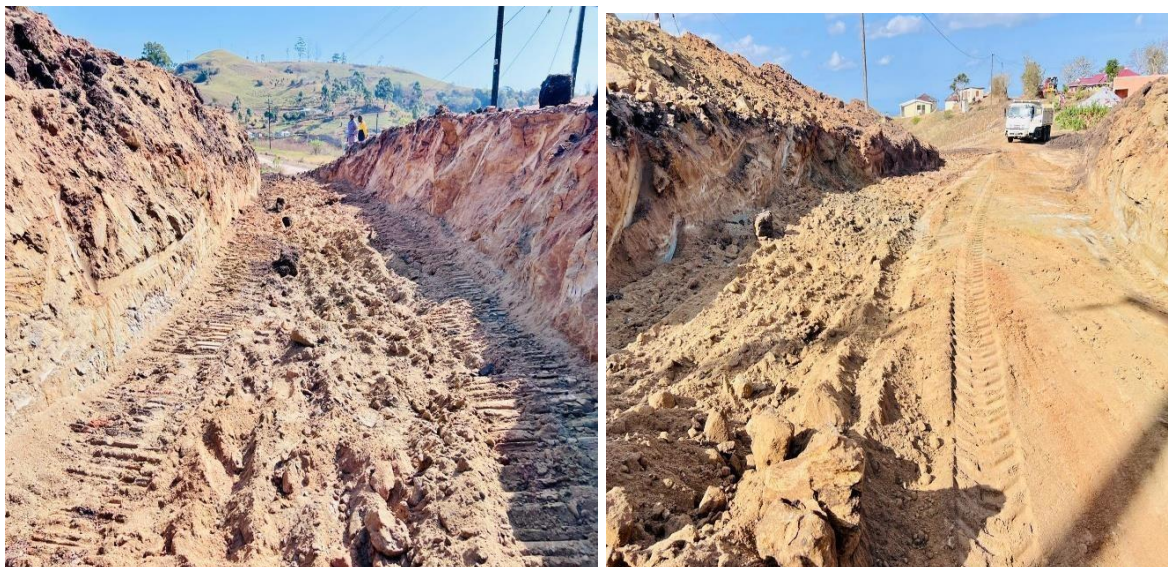
Photos: LIC Road Construction (Mqogha road, ward 09)
